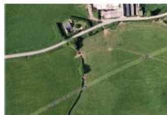
Site pre A477 construction (note gate access through fields)
